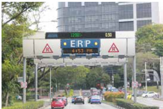
Figure 4-4 | Electronic Charging Gantry (left) and IU (right)
